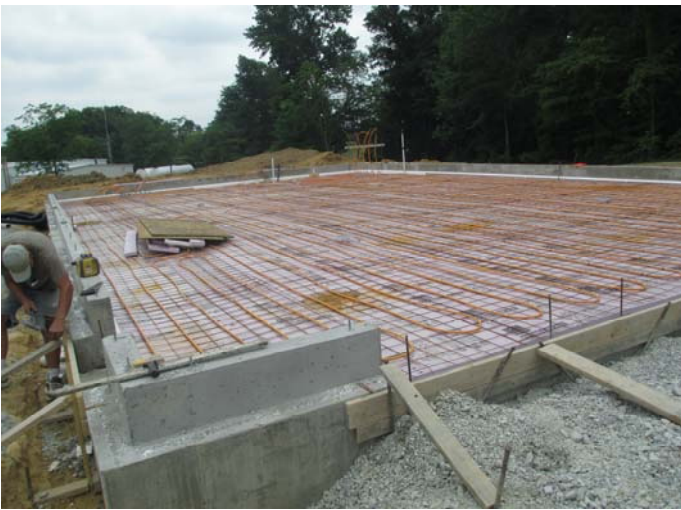
View showing the Radiant heat lines in the floor
