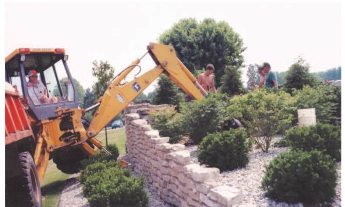
Maintenance digging the hole for the pole
