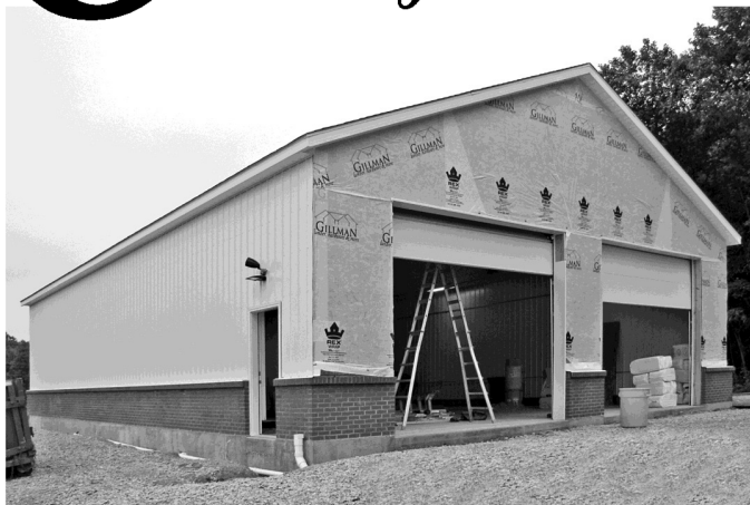
Clarksburg VFD Station #2 under construction at Lake Santee
