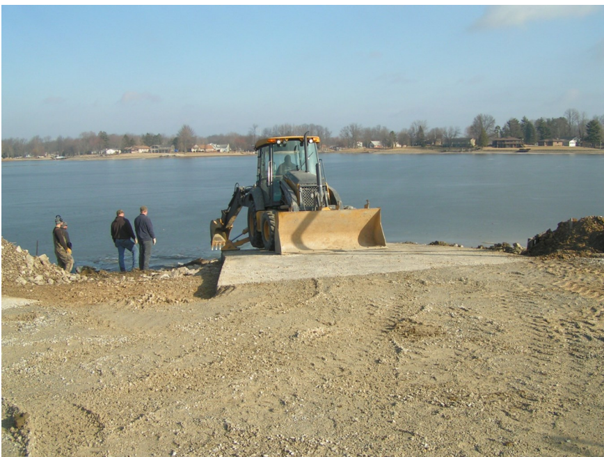
The Lake has been lowered 5 1/2 feet so that the boat ramps are exposed. The short steep ramp will be removed completely. The other ramp will have necessary
