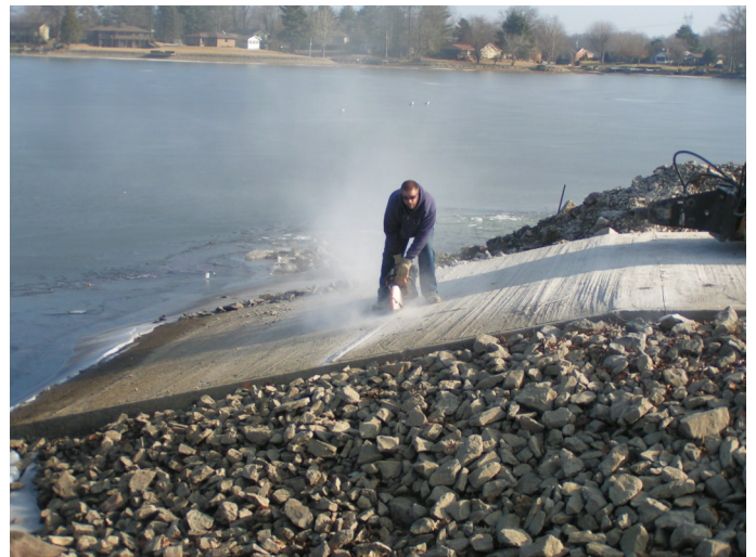
The Lake has been lowered 5 1/2 feet so that the boat ramps are exposed. The short steep ramp will be removed completely. The other ramp will have necessary
