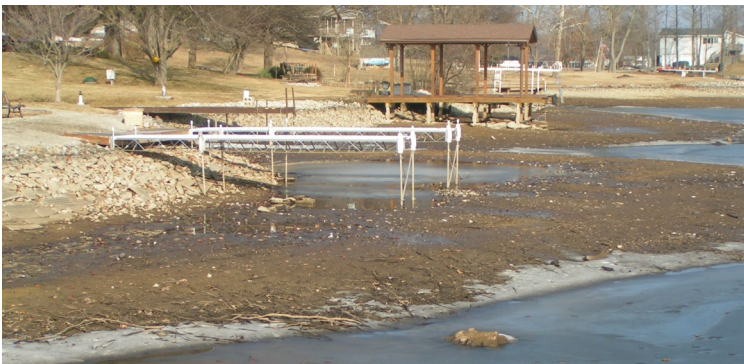
The Lake has been lowered 5 1/2 feet so that the boat ramps are exposed. The short steep ramp will be removed completely. The other ramp will have necessary
