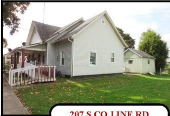
207 S CO LINE RD
