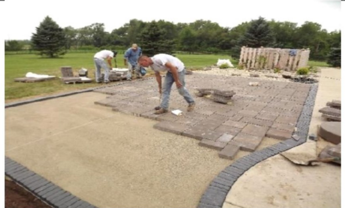
CONSTRUCTION IN PROGRESS
