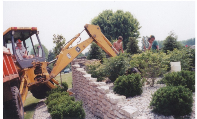
Maintenance digging the hole for the pole
